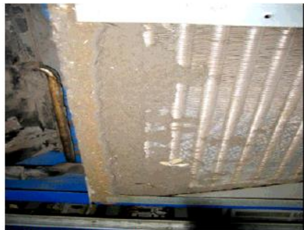
Clogged condenser coil.
